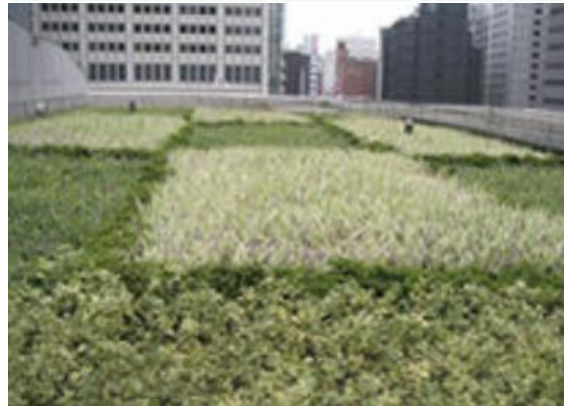
Rooftop greening (The Tokyo Metropolitan Assembly Building's rooftop)
