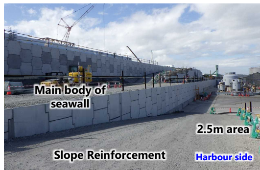
【Picture ①】 Main body of seawall under construction (2022.9)
