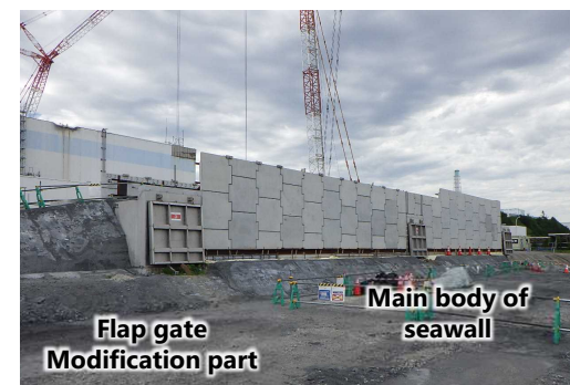
【Picture ②】 North side seawall under construction (2022.8)
