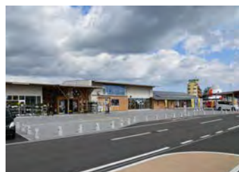
Namie Town: Roadside-Station "Namie"
