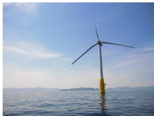
Floating-type offshore wind turbine in Goto city
