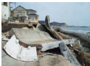
Iwaki City: Levee
