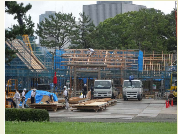
Daijokyu construction site
