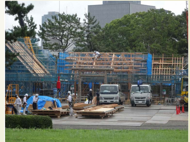
Daijokyu construction site
