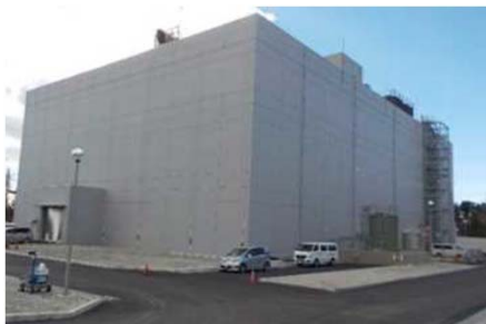
Miscellaneous solid radioactive waste incineration facility
