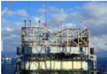
Unit1 : Removal of the cover was completed
