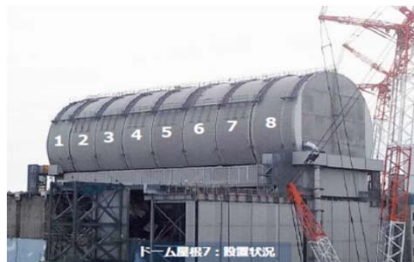
Unit3 Dome roof was installed
