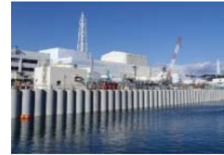
Sea-side impermeable wall
