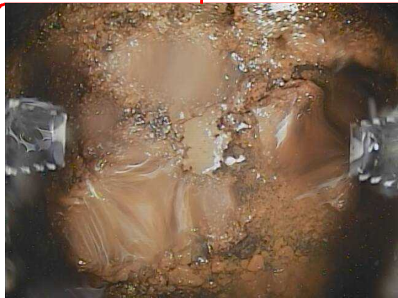
Before touching deposits
