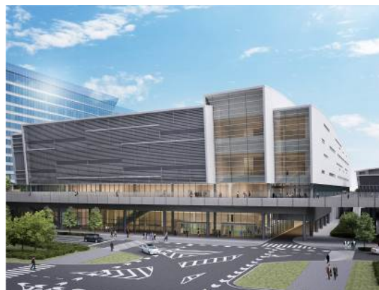
Exterior view of PACIFICO YOKOHAMA NORTH
