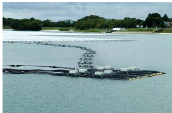
Power cables attached to solar panels
