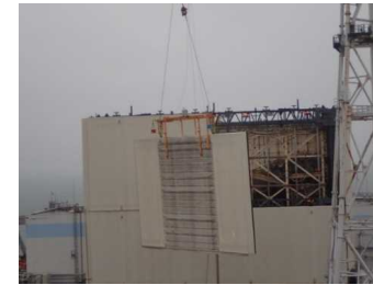
Removal of panels (Sep. 2016)
